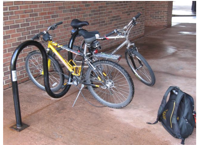
Front tire is exposed, which means it's easily bumped and can be damaged. Also, tire is not secured, and can be easily stolen.
